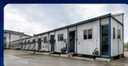
PREFABRICATED LABOUR COLONIES
